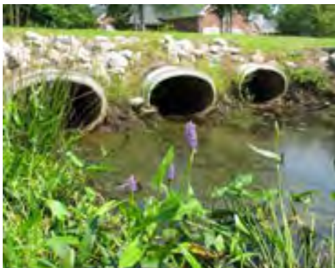
Inlet pipes convey stormwater from paved surfaces to the pond.
